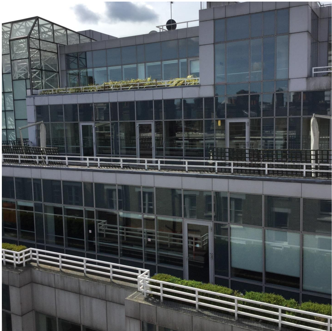
View of third, fourth and fifth floor terraces from Cecil Court
